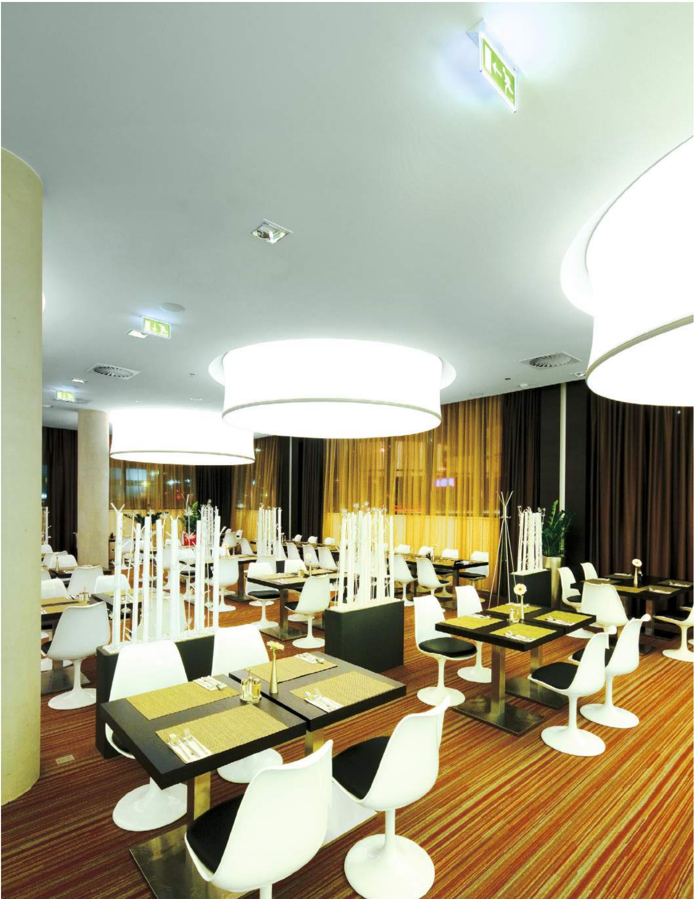
Hotel restaurant area emergency lighting application
