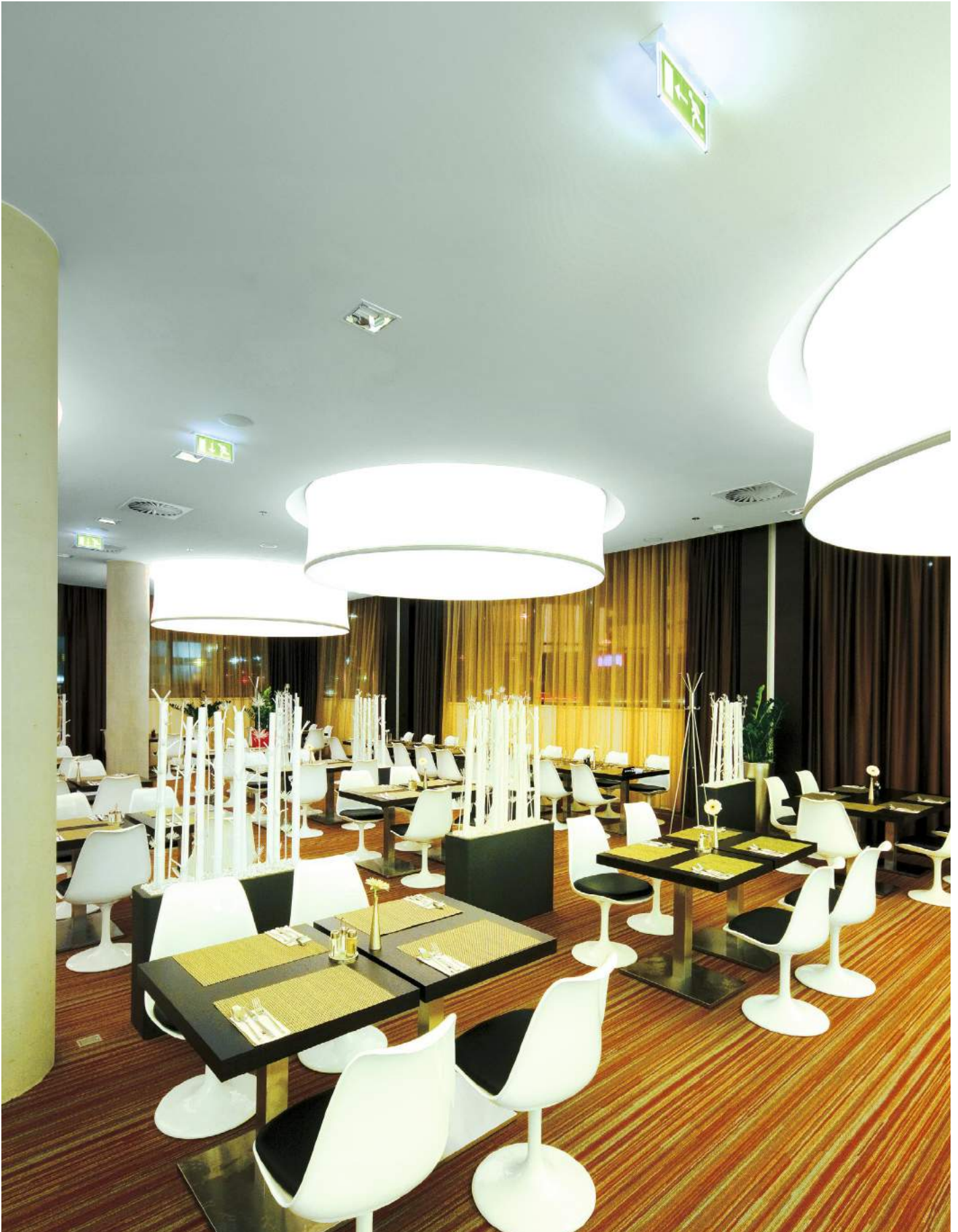
Hotel restaurant area emergency lighting application
